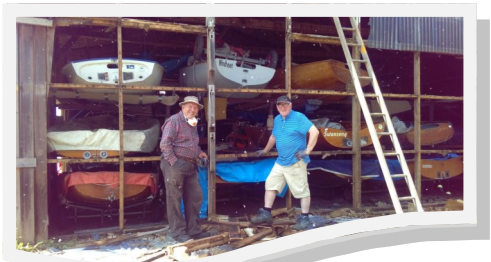
Peter and Liam have started work on the right hand side of the boatshed.
